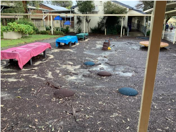
Photo 7: Example of hardstand adjacent to grassed areas, and planter boxes, photograph taken facing west (taken 05/07/2022).
