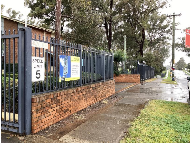
Photo 1: Main Access Gate (taken 05/07/2022).
