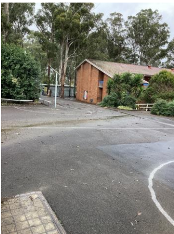
Photo 5: Example of school buildings and concrete playing court, photograph taken facing south (taken 05/07/2022).
