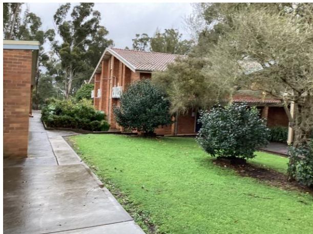
Photo 6: Example of school building, footpaths and grassed areas, photograph taken facing south (taken 05/07/2022).
