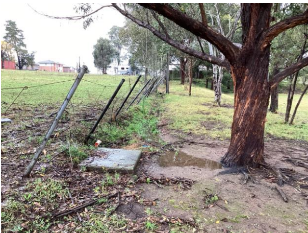
Photo 15: Example of stormwater pit located along the east perimeter of the field, photograph taken facing north (taken 05/07/2022).
