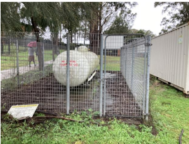
Photo 27: Photograph of above-ground tank, photograph taken facing east (taken 05/07/2022).
