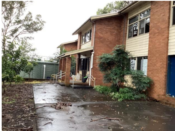
Photo 4: Example of school buildings, photograph taken facing east (taken 05/07/2022).
