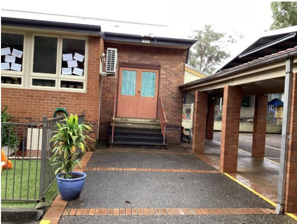
Photo 3: Example of school buildings, photograph taken facing east (taken 05/07/2022).
